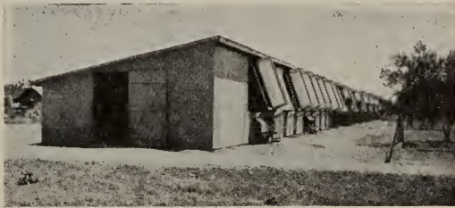
Fig. 55.—University type laying house containing five 40-foot sections and a 12-foot feed room at one end.
